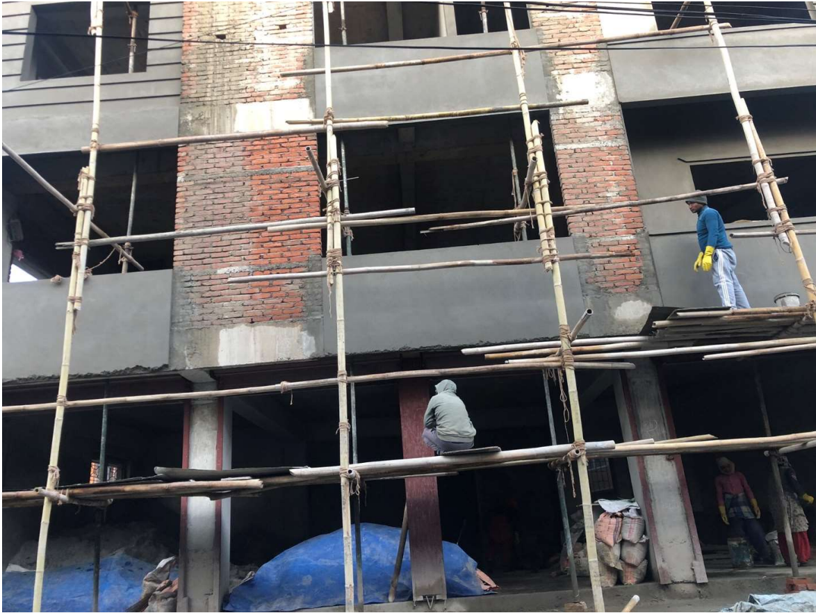
Figure 11: Site location (Dhapasi, Kathmandu), Cement used: Sarbottam
