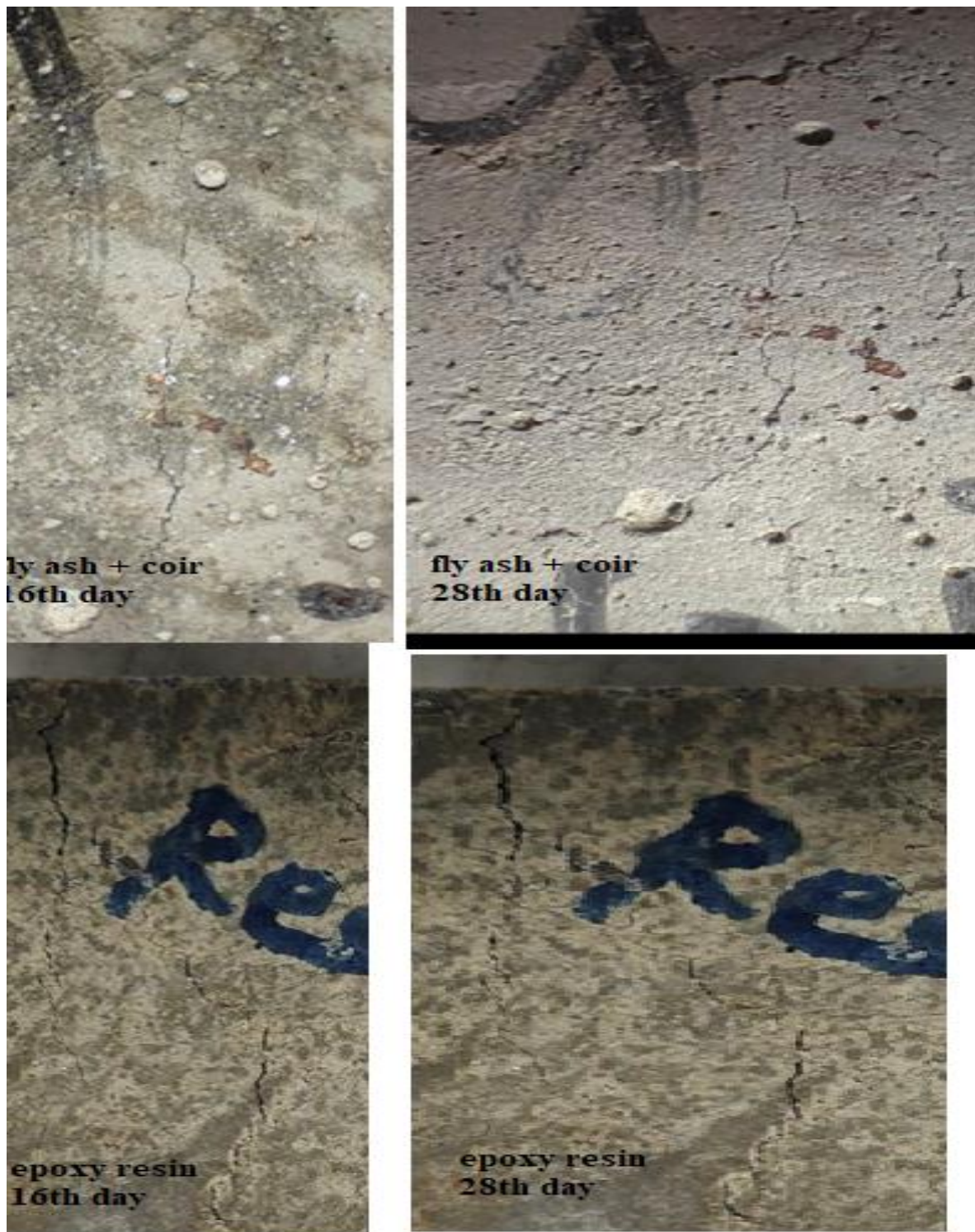
Figure 4: Visual observations of crack sealing of different mixes
